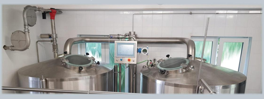
Fully automatic brewhouse brings safe and consistent operation. Brew master duty is focused to important technological checks, rather than operations what can be automated. Smaller batches allows more flexibility for different beers. In case of larger brewhouse, main obstruction is transportation of oversized cargo what become very expensive. On site construction of pans is also not an option as that also create excessive costs and jeopardize finish of pans.
