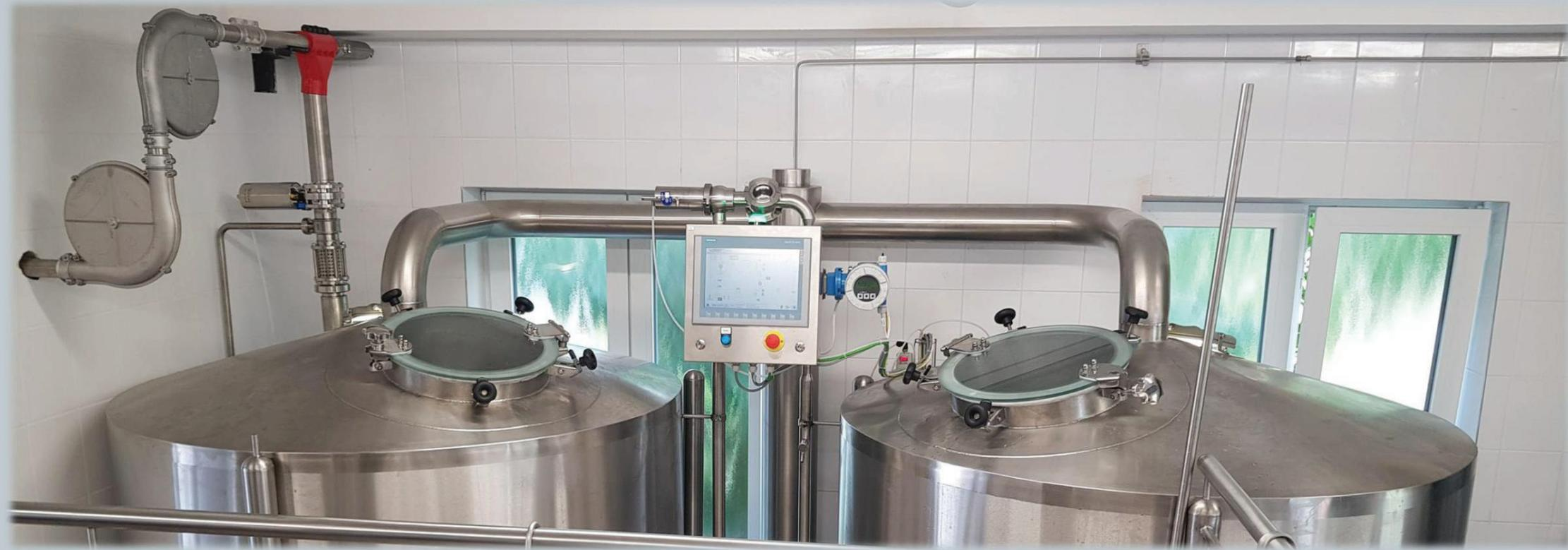
Fully automatic brewhouse brings safe and consistent operation. Brew master duty is focused to important technological checks, rather than operations what can be automated. Smaller batches allows more flexibility for different beers. In case of larger brewhouse, main obstruction is transportation of oversized cargo what become very expensive. On site construction of pans is also not an option as that also create excessive costs and jeopardize finish of pans.
